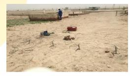
Pipeline Current Mapping Survey (PCM)
